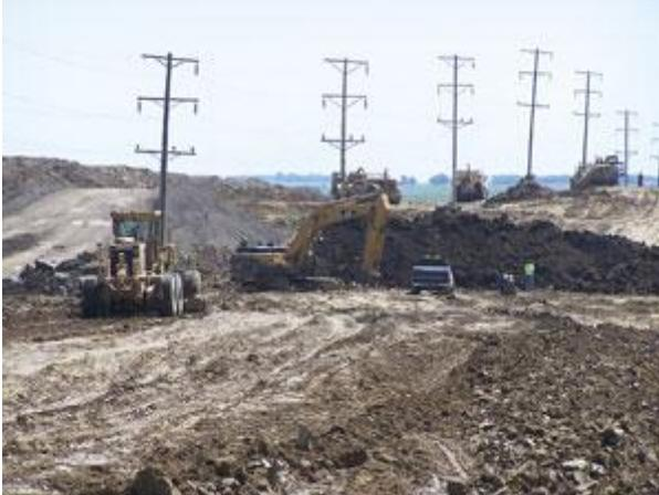
R & G Construction excavated areas to install concrete storm sewer pipes before grading the highway.
