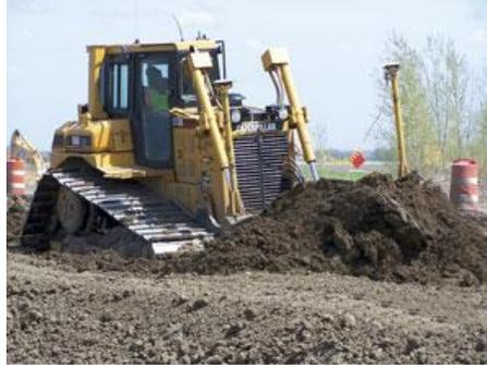
**A Caterpillar D6R dozer with GPS moves along the sides of Highway 34 as it levels the road.**
